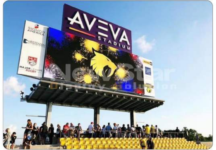
STADIUM PROJECT IN HOUSTON
